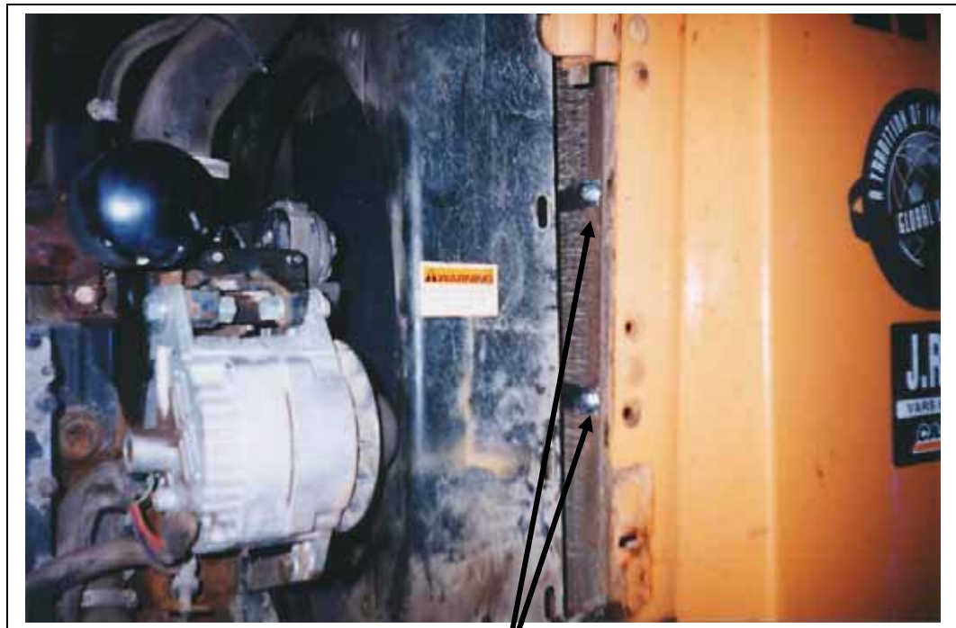
Condenser brackets on left side of radiator
